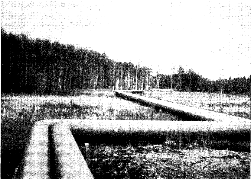
Fig. 47: Expansion bend in a district heating line.
